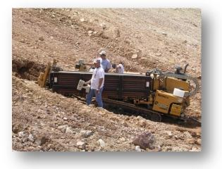
cobbles, it was necessary to drive steel casing to an intermediate depth of approximately 30 feet and then continue the boring to the total depth. PVC pipe was then inserted to the total depth of each well.
