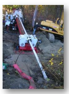
drill head designed for these extreme soft conditions, the borehole was advanced to the next soil
