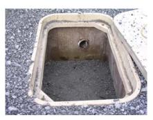
near horizontal well screen. The vault has to be designed so pumps and other tools can slide into the well without snagging on the vault. Engineers must examine the length of the pumps and instrumentation to ensure it fits within the vault.
