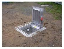
Below ground horizontal well completions are similar to vertical well completions in that they use vaults, but the similarity ends there. Horizontal vaults have to accommodate the
