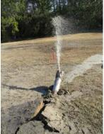
Once the drill head has reemerged at the surface, it is removed from the drill string and replaced with a reamer. The reamer is designed to enlarge the borehole to accommodate the well materials. Typically the well materials are attached directly behind the reamer and pulled into the borehole.
