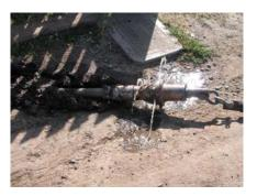
Sometimes the reamer is pulled through the borehole one or more times to enlarge the hole or condition it to make the pull back easier.
