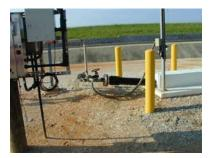
Horizontal wells offer other challenges once they have been installed. Since they exit the ground at an angle, traditional completions are not appropriate. Like vertical wells, they can be
