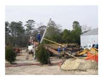
The locating technician typically does not come near the entrance or exit pits. This person walks over the drill head, noting its location and orientation. Unless the ground surface is contaminated, this person rarely comes into contact with contaminated materials. The laborer who assists with pumping the pits and attaching the various drilling tools usually comes into contact with contaminated materials. This person, and anyone who may work with them in the pits, will often require PPE.
