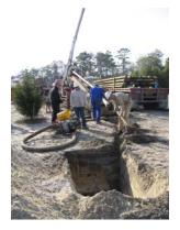
Larger drilling rigs typically do not have automated rod loaders. These rigs usually load the drill rods with a crane, requiring additional workers and the risks associated with heavy loads overhead. The drill rods typically are brought to the rig on a trailer and there are issues with working above ground without a place to tie off.
